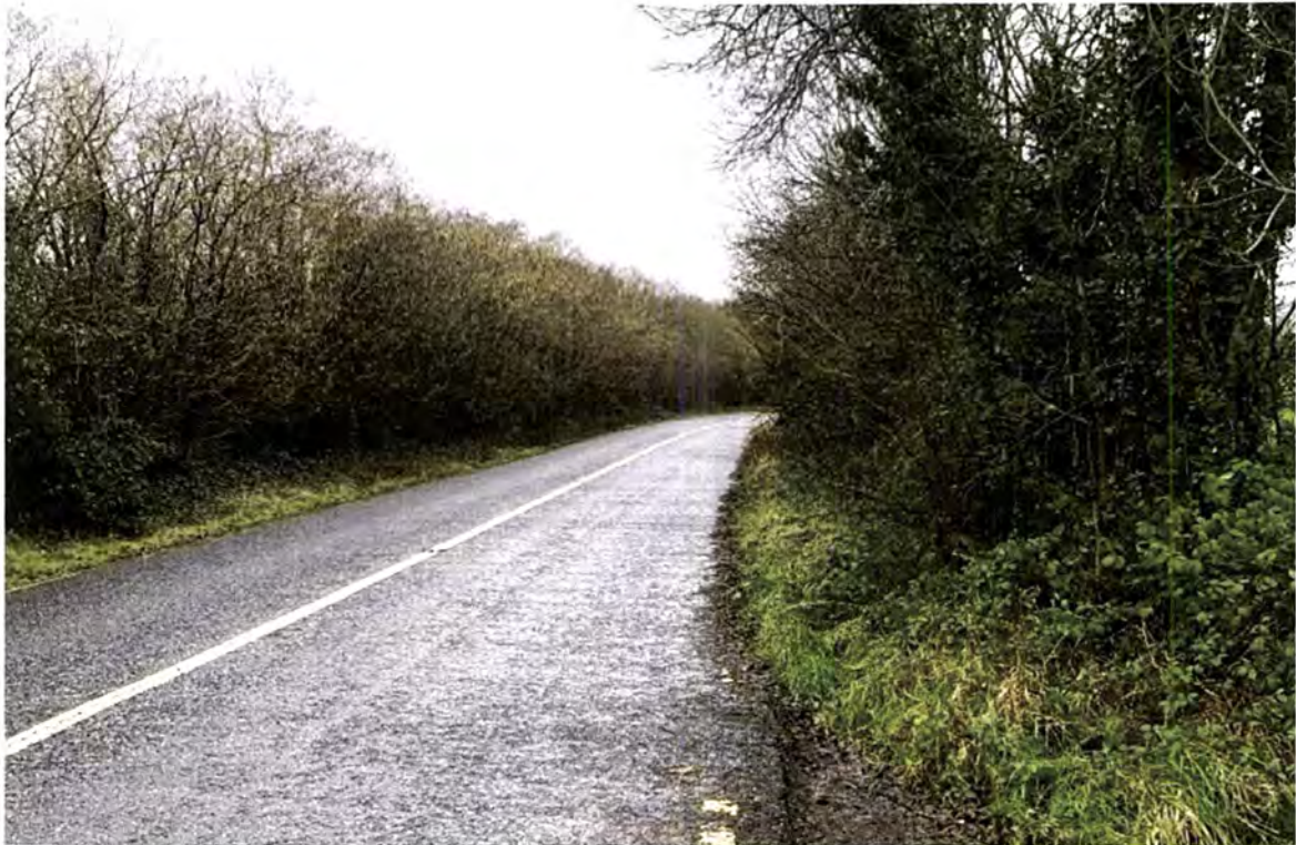
Plate 2: R772 at access point into adjacent field.
